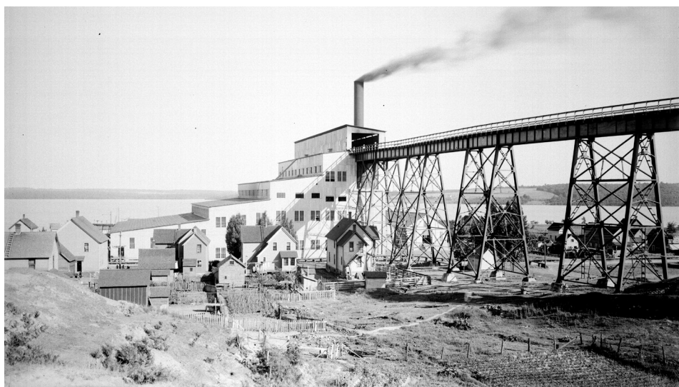
Photograph of Ahmeek stamp mill located in Tamarack City, Michigan. Photo provided by the Michigan Technological University Archives and Copper Country Historical Collections.
