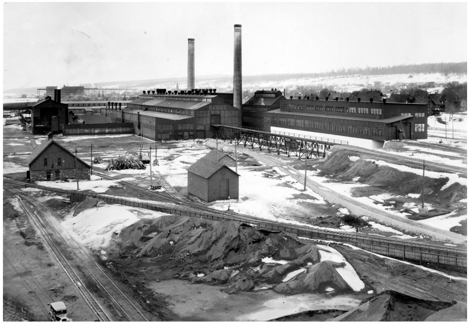
Photograph of C&H smelter and concentrate storage building in Hubbell, MI about 1950. Photo provided by the Michigan Technological University Archives and Copper Country Historical Collections.
